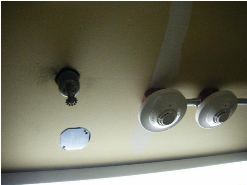
Example of "Sprinkler and Smoke Detectors"
