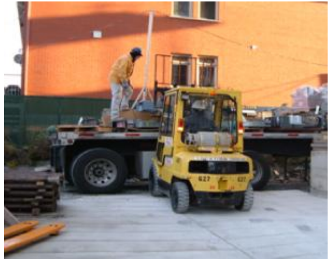
Example of “Use of Forklift” (Forklift Provided by Others)
